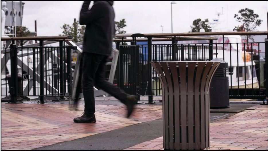
Figure 2: Example of 5G antennae in dust-bin cover (Auckland).
