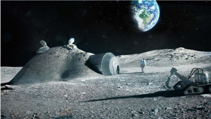
Fig. 5.1 Representation of a module of a lunar village (Credit: ESA/Foster + Partners). The dome is protected from radiation, temperature variations and meteorites thanks to a layer of regolith. Outdoor light could be collected via special windows through the regolith-based protective layer. The village is a network of modules linked together by tunnels
