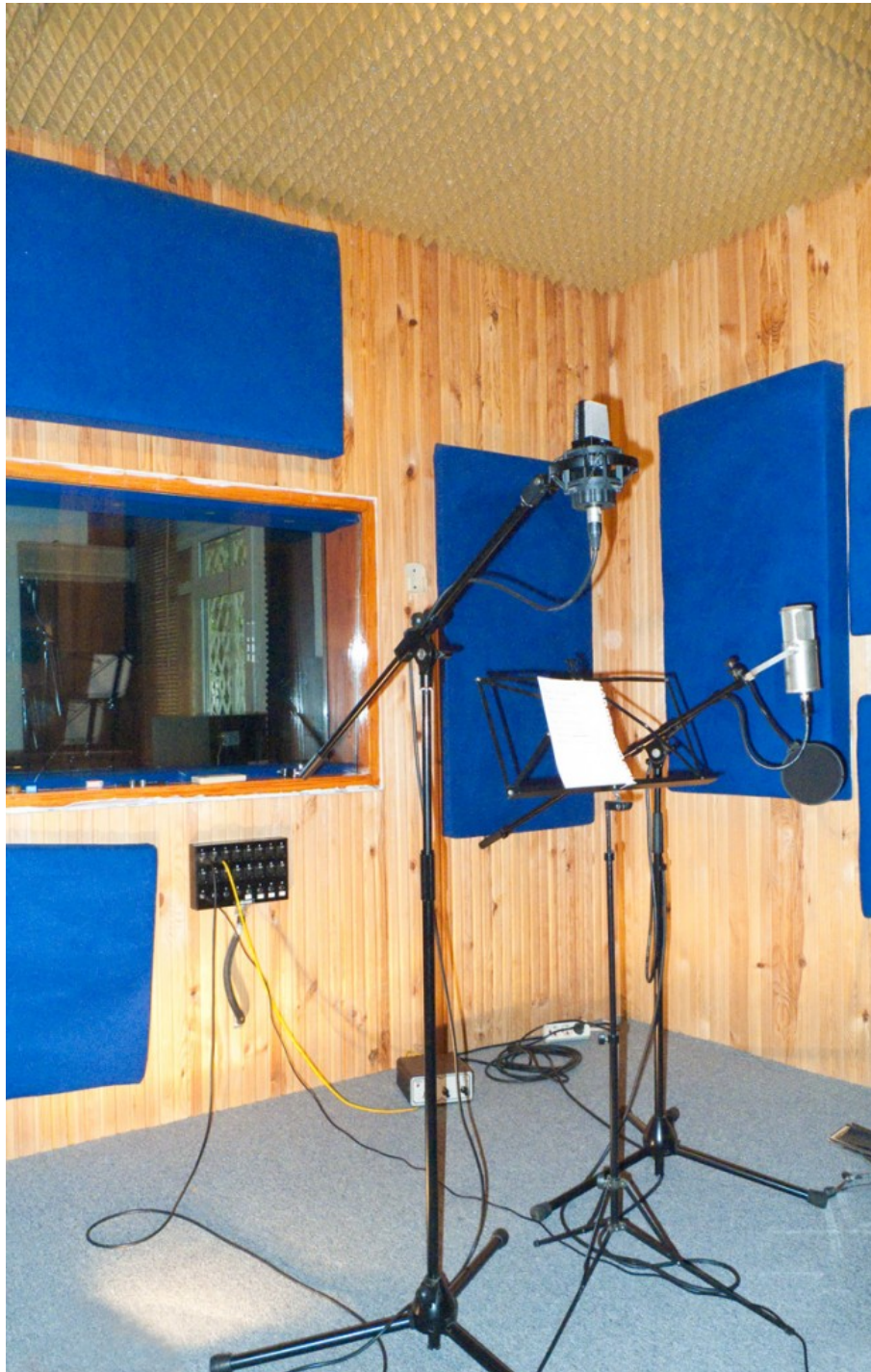
Figure 6. Broadband absorbers hanging in the tracking room at Duru Kayıt, İstanbul.
