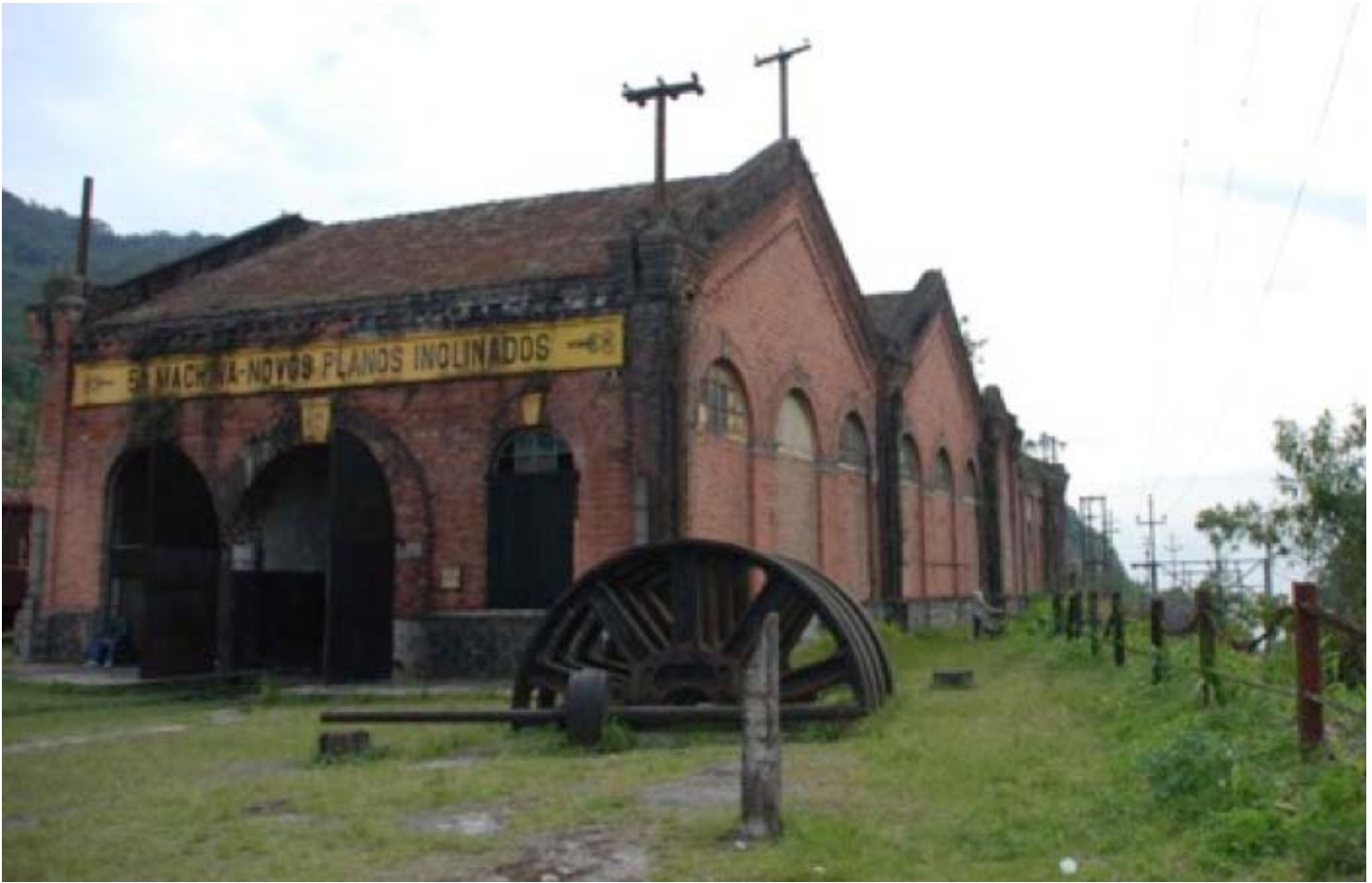
Railway shed containing the 5° Stationary Steam Engine, New Inclined Plane designed by the engineer Emilio Schnoor and built by the São Paulo Railway (1895-1902). Photo: Eduardo Romero de Oliveira.
