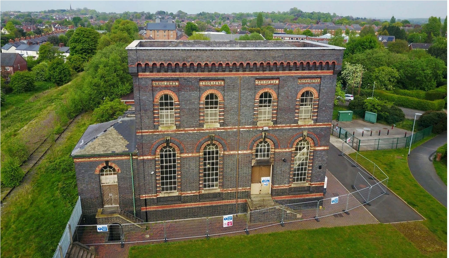
The 1874 engine house is mostly of blue engineering bricks with coloured brick decoration.
