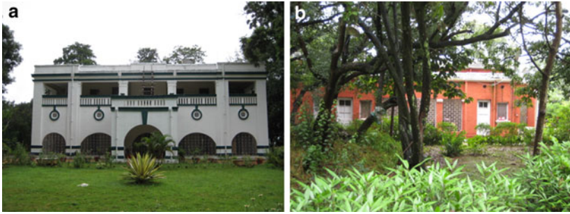
Fig. 1 Superintendents' residences: a Berkeley-Hill, European Mental Hospital b Dhunjibhoy, Indian Mental Hospital (Author's photographs 2009)
