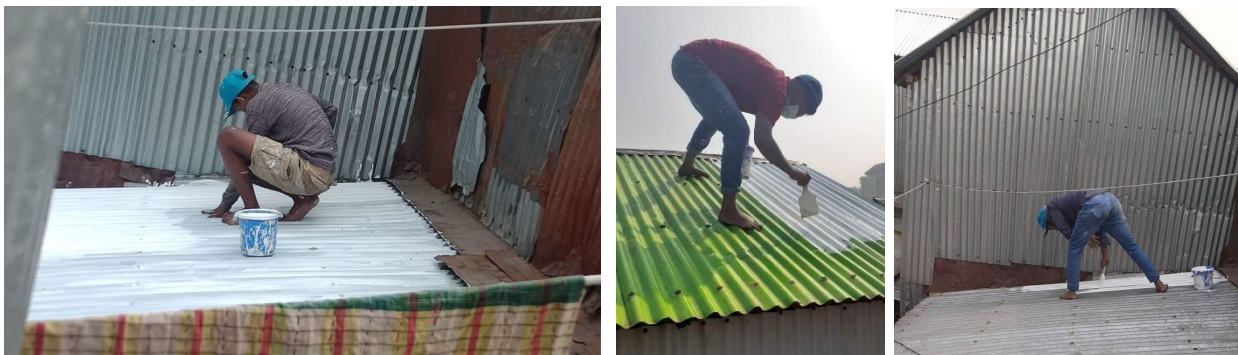
Figure 6: Cool roof coating application. Source: Authors
