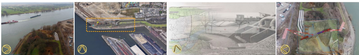
Figure 1: Site view of the estuary area of the new post-industrial park (left two images), digital twin for the bridge (middle), and assembly location for the bridge (right). Source:(©Thomas Spiegel2022).
