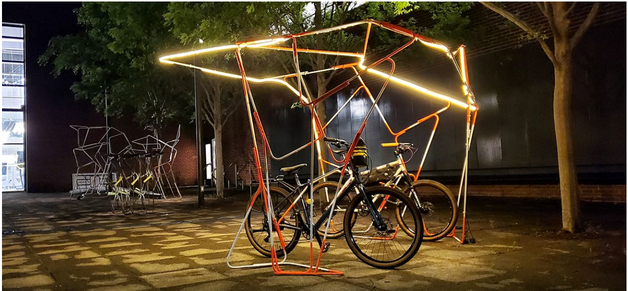
Figure 6: Final installation of the bike shed designed and produced through MR in twenty person-hours. Source: (SFL 2022)
