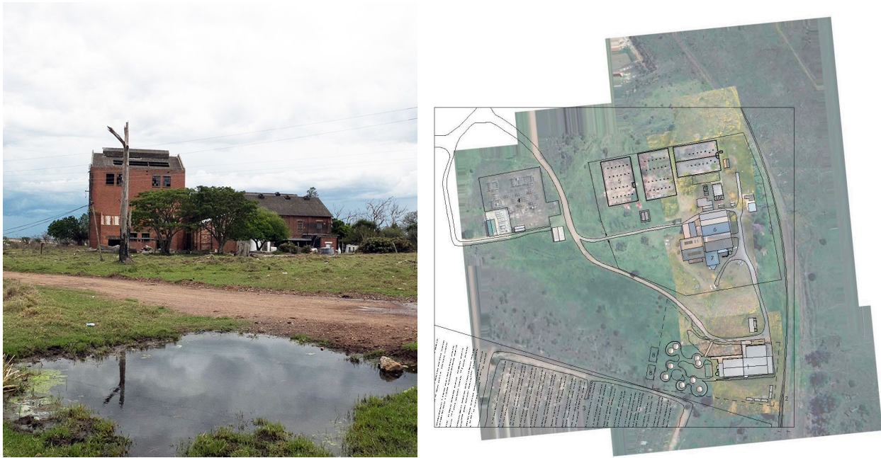
Figure 2: View and site plan of The Black Power Station. Source: Crisman studio 2022
