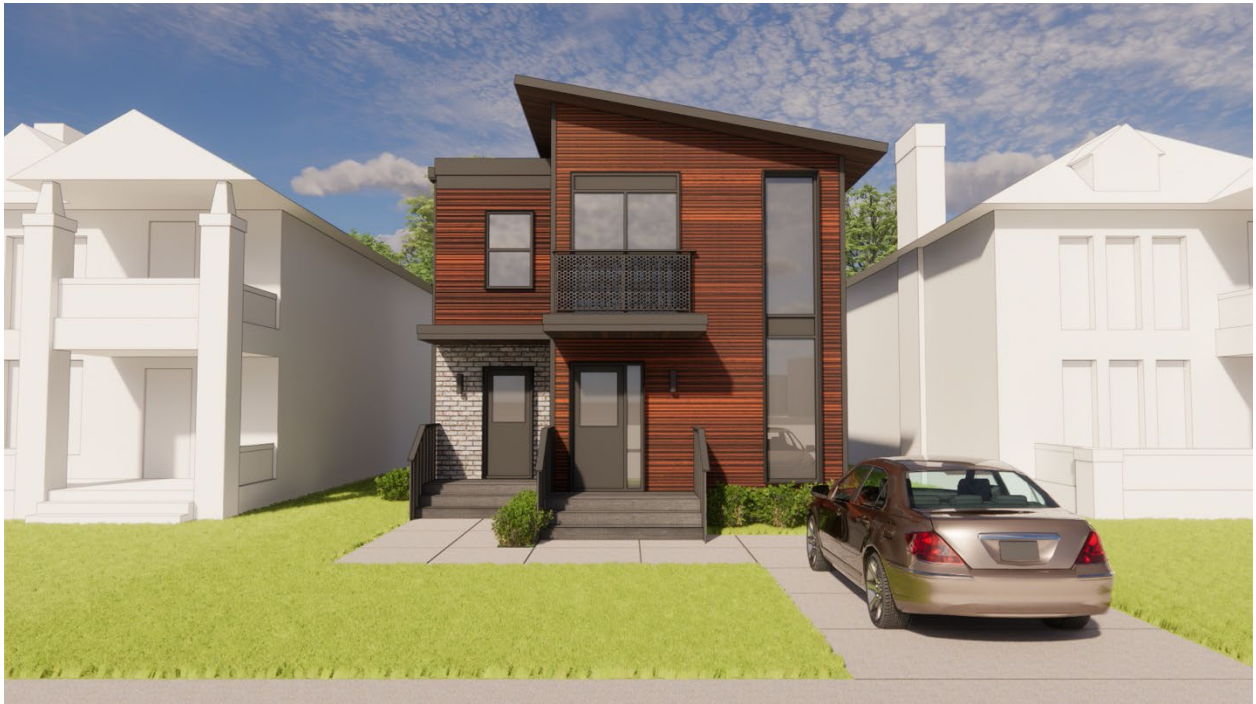
Figure 5: The Elmhurst Duplex by Three Squared International leverages the use of reclaimed shipping containers to reduce the cost and time needed for construction. (Image courtesy of Three Squared International.)
