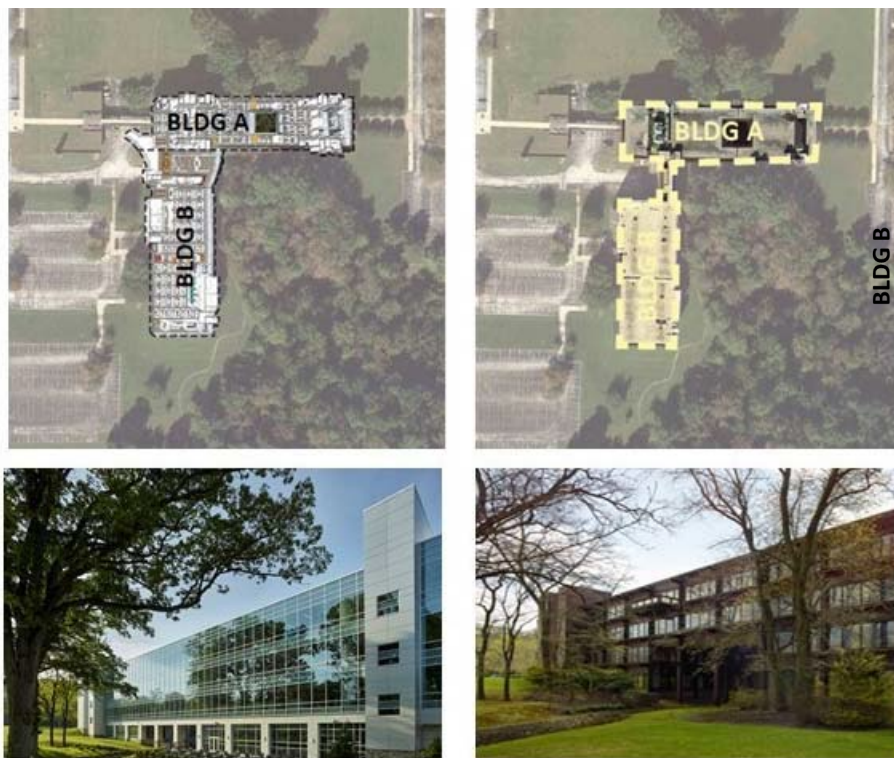
Figure 1: The building complex before (right) and after retrofit (left). Source: Author 1
