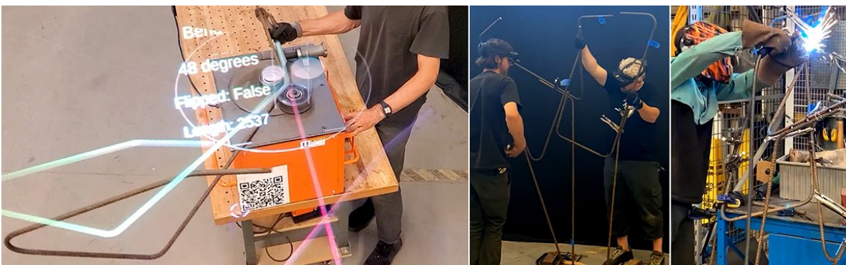
Figure 5: MR-assisted rebar fabrication workflow: holographic bending, assembly, and final welding. Source: (SFL 2022)
