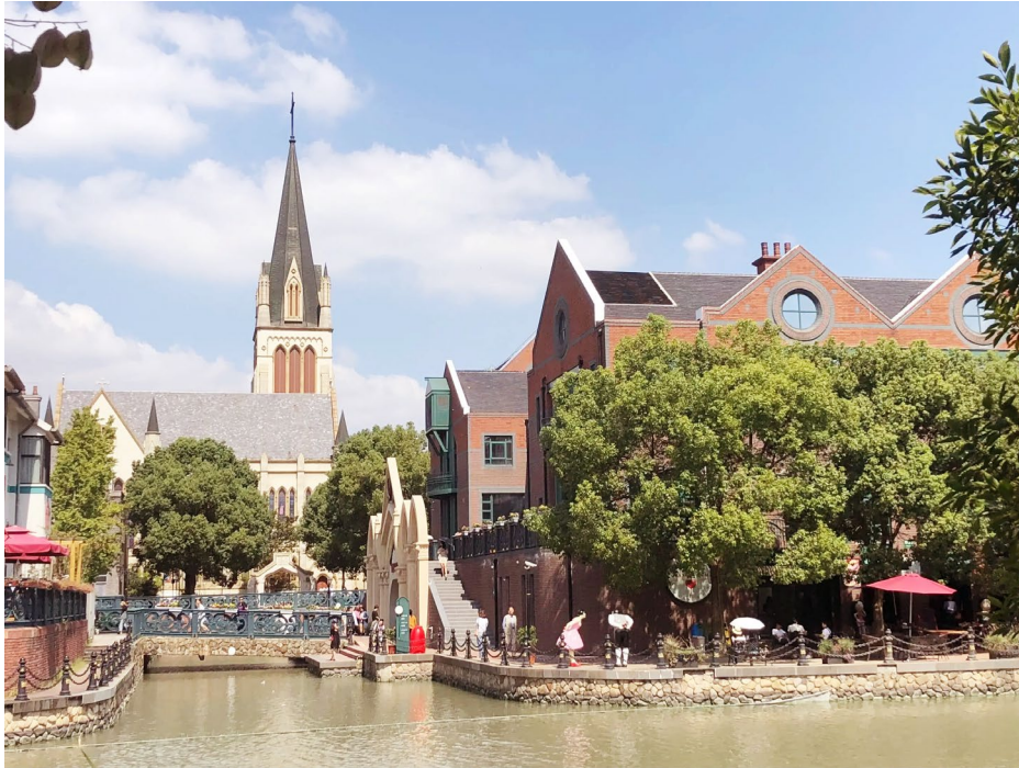
Figure 3: Buildings within the Thames Town borrow architectural forms from different British styles in history. Source: (Author 2019).
