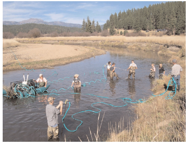
Fig. 2. Volunteers are sometimes enlisted to use equipment for facilitating planting along riverbanks. In this initiative a waterjet stinger is being employed (Kent Werlin) (By permission of photographer Kent Werlin)
