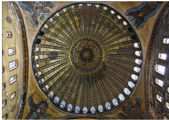
Figure 1: A view of the central dome of Hagia Sophia from below. Note the small irregularity of the upper cornice. Note that the foundation of the dome springs directly from the upper cornice. Source: https://www.flickr.com/photos/ficablok38/8432896767
