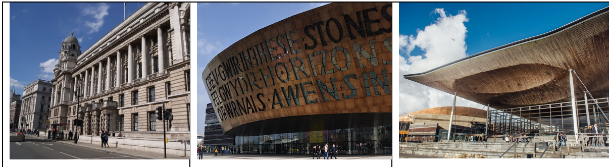
Left (figure 107) The Old War Office, Whitehall; Middle (figure 108) The Wales Millennium Centre, Cardiff; Right (figure 109) The Senedd, Cardiff
