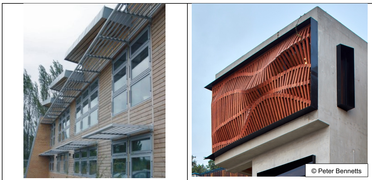
“Reduce heat gain”: Left (figure 75) Functional brise soleil; Right (figure 76) Sculptural brise soleil
