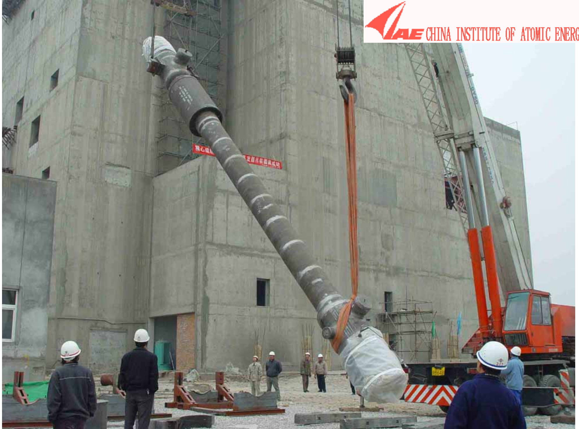
Evaporator Moving to Reactor Building (2005.03)
