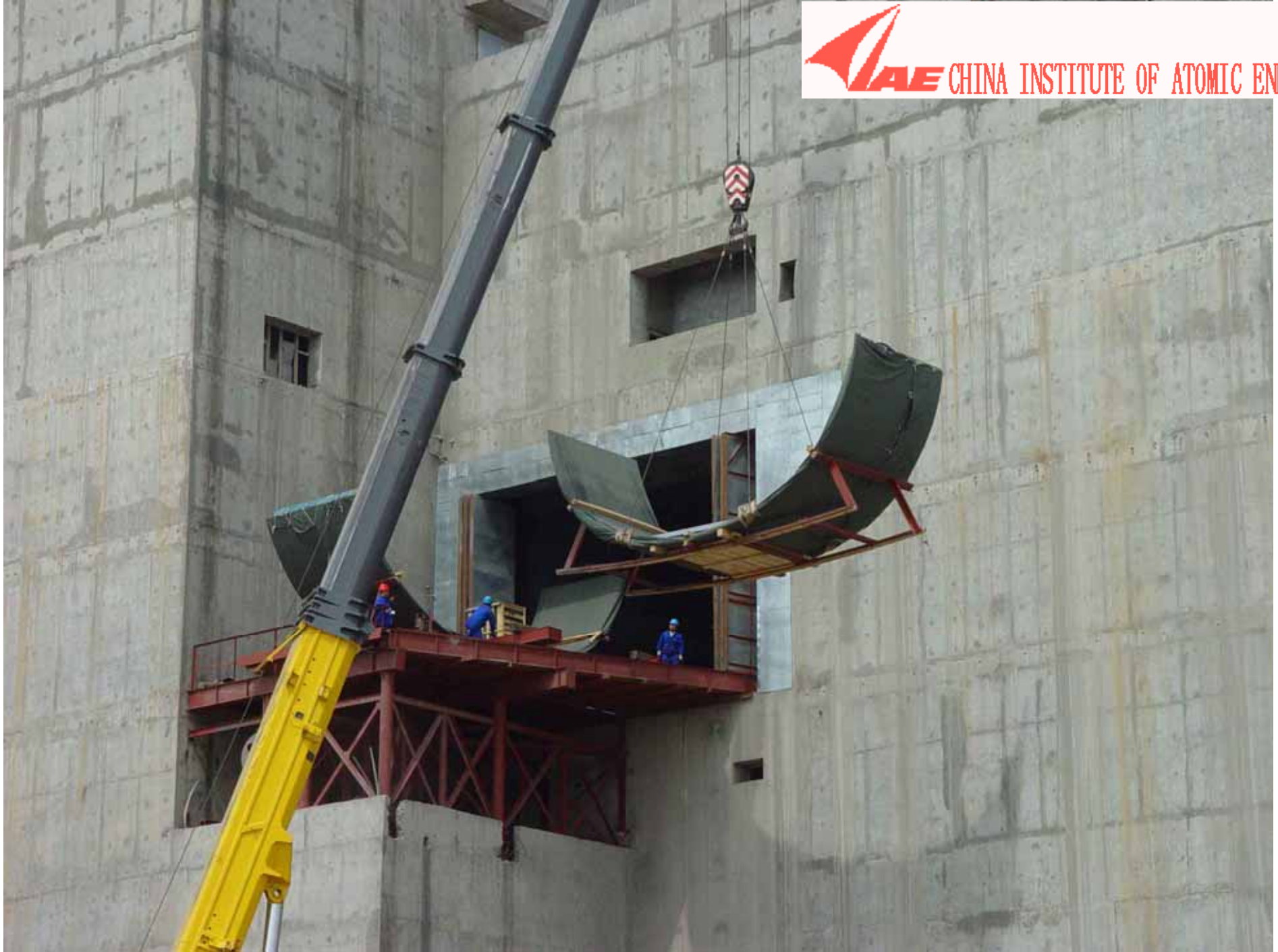
Some Parts of CEFR Main Vessel Moving to Reactor Building (2005.04)
