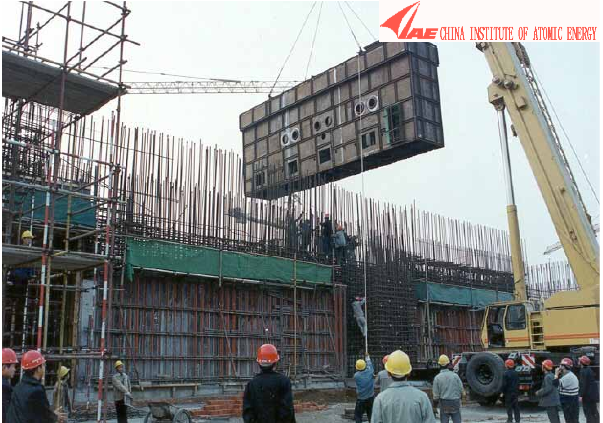
CEFR Hot Cell under Installation (2001.10.26)
