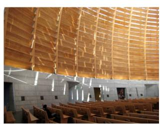
FIG. 4 INTERIOR VIEW OF CONCRETE RING AND WOODEN VAULT IN DOUGLAS FIR
