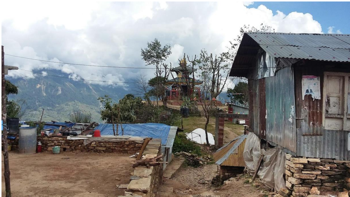
Figure 5.7. Buildings in Listi in the foreground, using brick and corrugated galvanised iron sheets and in the background, timber frames on brick (Photo credit: author, 2017).
