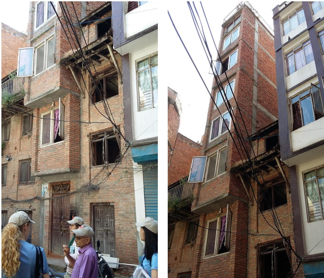
Figure 5.9. Some examples from the NSET Vulnerability Tour, highlighting buildings that are particularly vulnerable to earthquakes (Photo credit: author, 2017).
