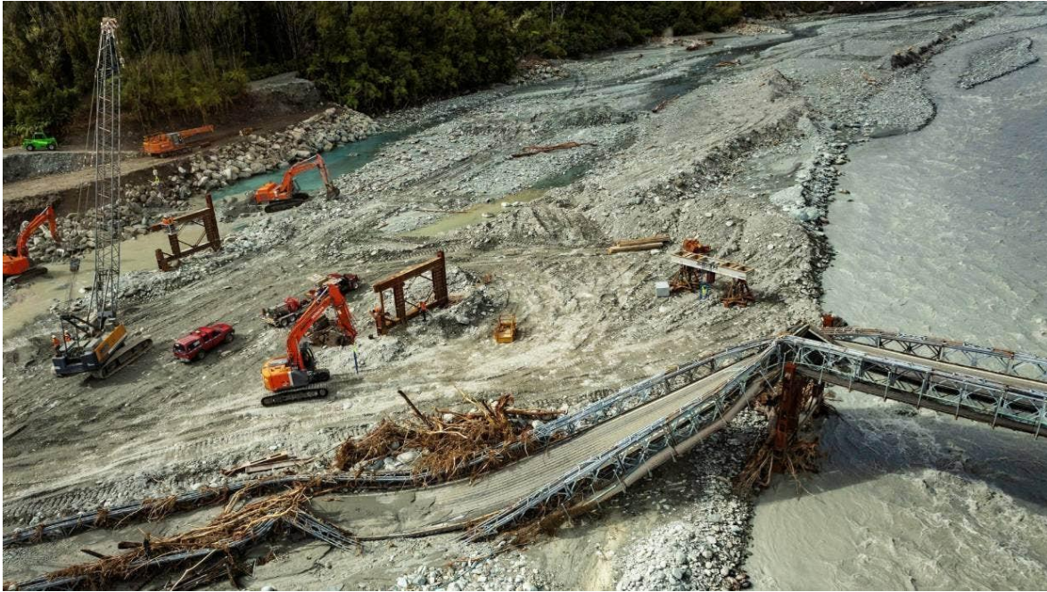
Figure 6.5. The aftermath of the flooding which wiped out the Waiho bridge (Photo credit: Stuff NZ).
