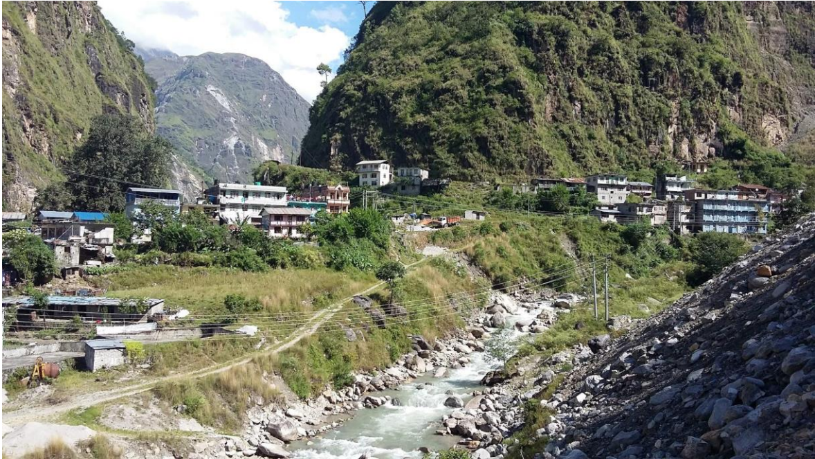
Figure 5.2. Approaching the settlement of Larcha with landslides prominent (Photo credit: author, 2017).
