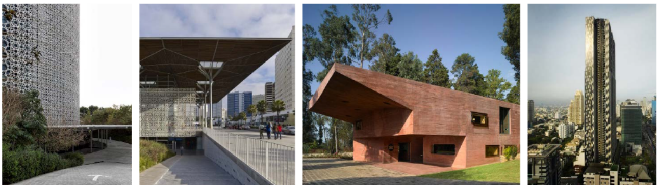
Figure 3. Doha Tower (Doha, Qatar); Casa-Port Railway Station (Casablanca, Morocco); Embassy of the Netherlands (Addis Abeba, Ethiopia); The Met Tower (Bangkok, Thailand) (right to left)
