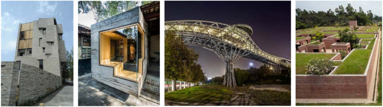
Figure 1. Apartment No. 1 (Mahallat, Iran); Micro Yuan'er Children's Library & Art Center (Beijing, China); Tabiat Pedestrian Bridge (Tehran, Iran) and Friendship Centre (Gaibandha, Bangladesh) (source: on site review reports, Aga Khan Award Cycle 2013–2016) (right to left)
