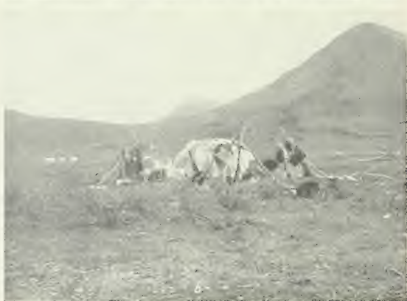
A dome-shaped willow hut at northwestern entrance to Anaktuvuk Pass, Alaska. a , Hut being erected. The poles in foreground were imported from south of mountain divide. A radio aerial is seen to the right. b , The same hut finished and covered with caribou hides. In the background are store-bought tents of other Killik Eskimos.
