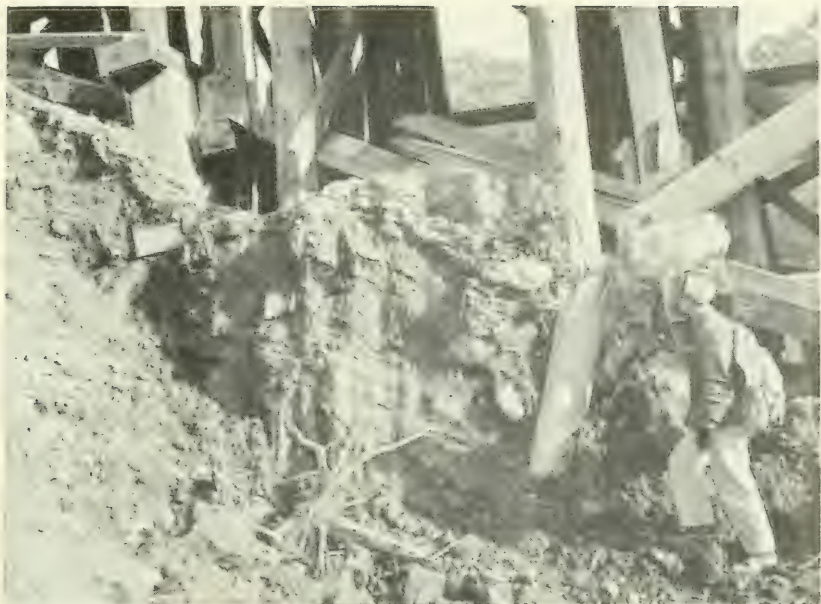
1. Bridge piling on the Alaska Railroad broken by downhill creep in mud on top of permafrost in the Nenana River Gorge, central Alaska. Photographed September 24, 1948.
