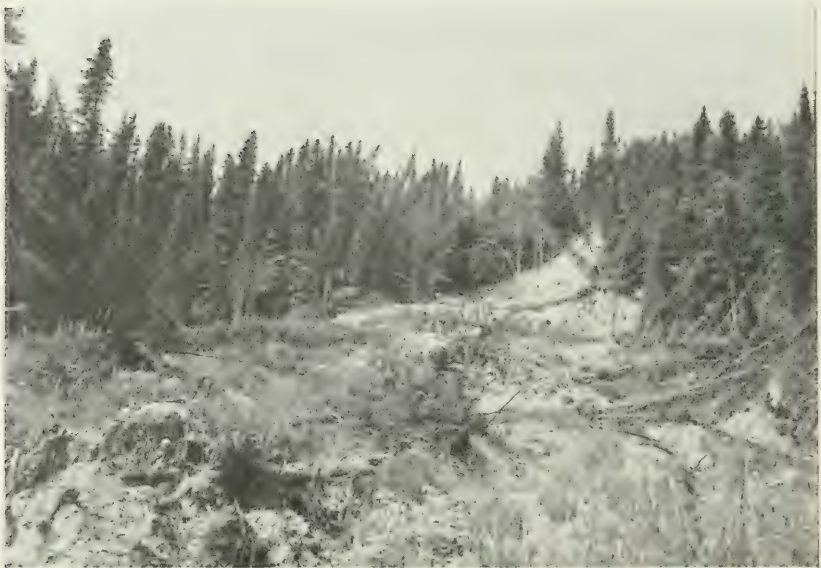
2. Landslide on top of thawing permafrost on Slana-Tok Cut-off, 27.9 miles from Gakona in east-central Alaska. Photographed July 9, 1946.
