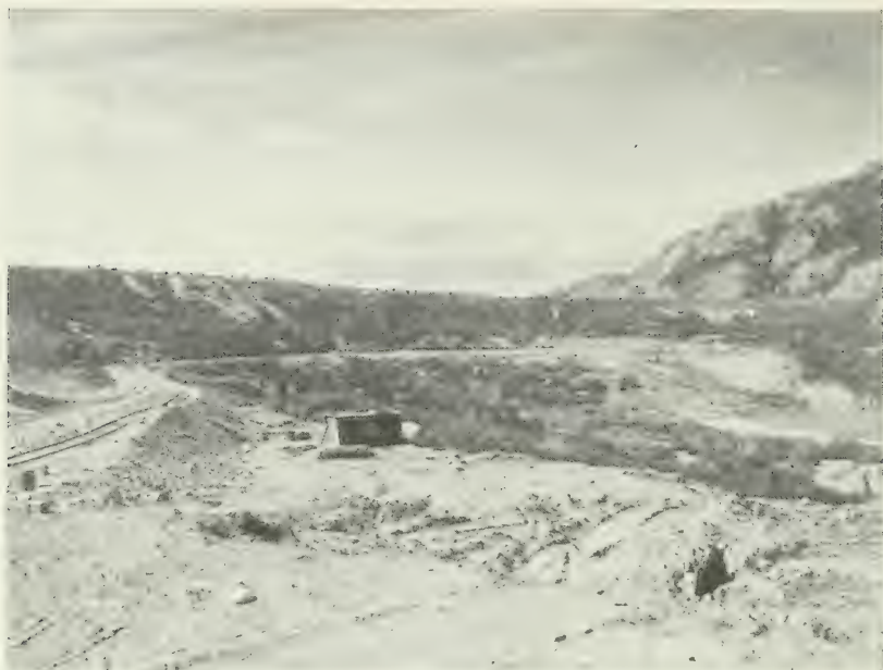
1. Mud flow on top of permafrost along the Alaska Railroad resulting in track settling, near Moody, Alaska. Photographed June 22, 1948.
