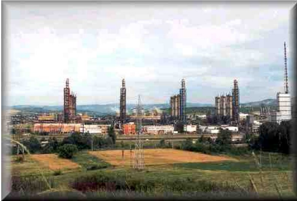
Figure 4. Heavy Water Plant - Overview. Source: ROMAG website
