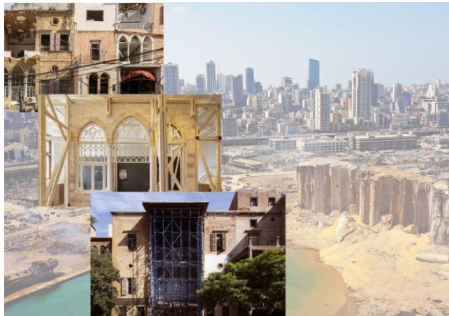
Figure 1. The blast of the container in the port of Beirut and the dramatic consequences on historical buildings.
