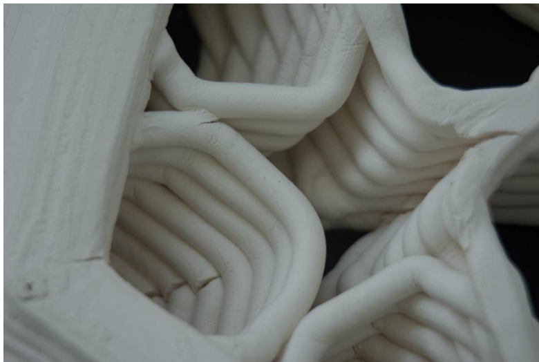
Figure 7: Cracks observed in interior walls of ‘shrinking’ prototype print, caused by differential thickness and drying time between interior and perimeter walls.
