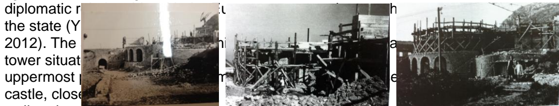
Figure 10: The entrance to the citadel, museum under construction (Institute of Cultural
