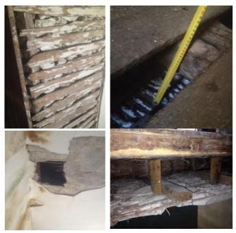
Fig. 4. A. Wooden indoor partition wall; B. Wooden slab; C. Bottom cover of the wooden slab; D. Section of the wooden slab Source: K.Xhexhi
