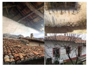
Fig. 5. A. Wooden roof; B. Outer stone wall; C. Ceramic tiles of the roof; D. Concrete pavement connected to the ground floor Source: K.Xhexhi
