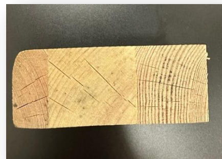
Figure 2. Changes on the wooden surfaces of elements. Source: Authors
